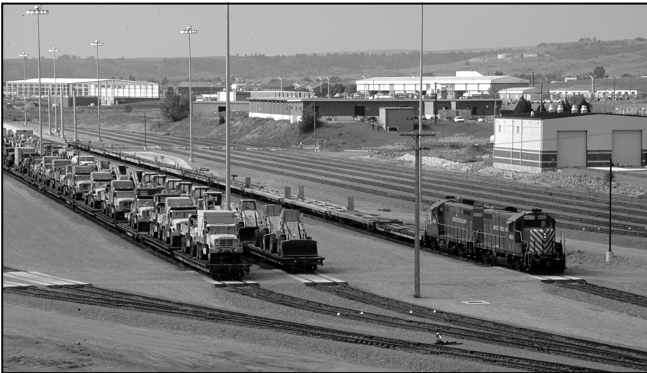
U. S. Army GP-16's 4633 and 4628 were switching the new stub end load/unloading tracks at Fort Carson's Railyard on 6/20/01. Above the red and yellow Army switchers is the new two-stall engine house, which was still under construction. – Photo © Chip.
