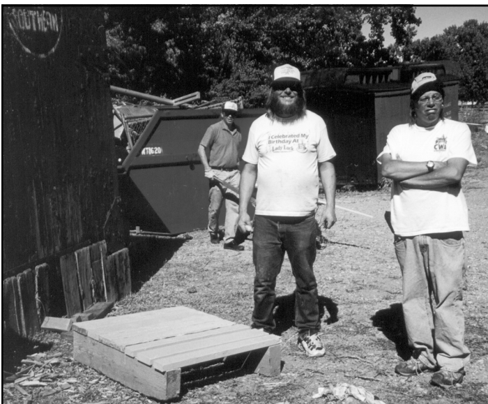
Matt and Mark Tomon rebuild and repaint steps while Ken Gow hauls trash. – Photo © Bob Tully.
