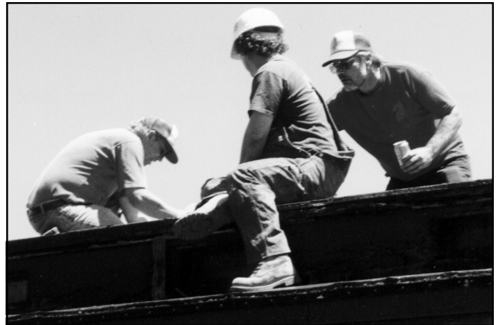
Ken Gow, Bill Kepner and Dwane Fields scrape the roof and apply roofing tar to the roof of the Rico prior to painting. – Photo © Bob Tully.
